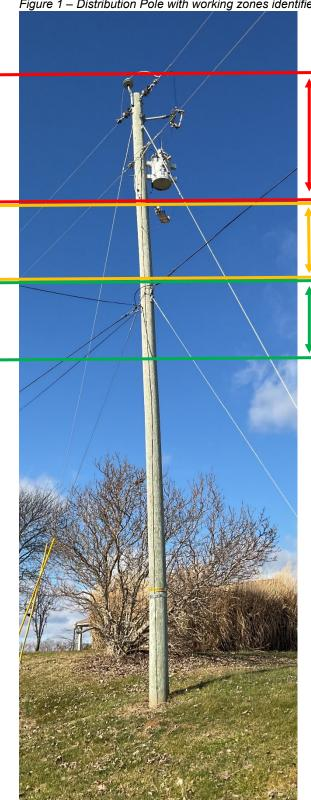
Power Supply Space – reserved for electric distribution use. Communications attachments and unqualified workers should not be in this working zone on the pole.
